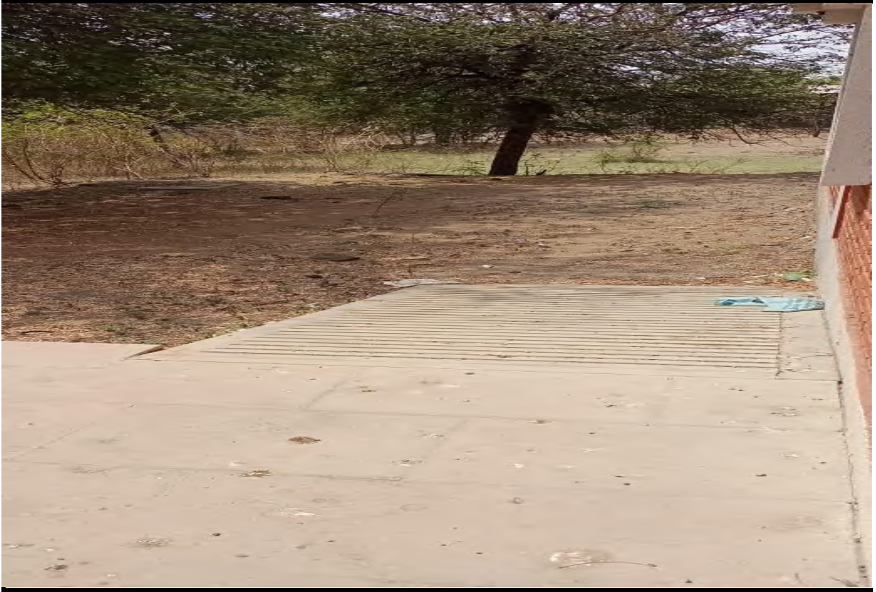
Wheelchair Users Ramp
